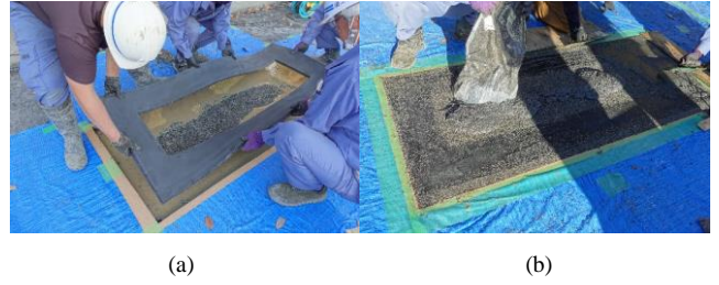
Fig. 13. Embedding process of thick case coil. a) Coil setting. b) Coil embedding.
