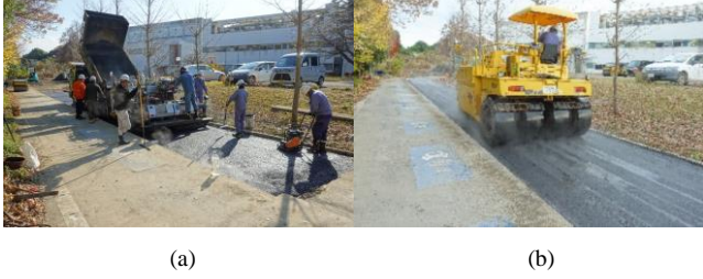
Fig. 9. Asphalt repaving situation. a) Laying asphalt. b) Rolling compaction.
