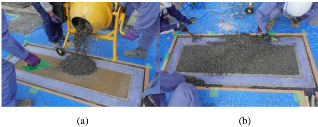
Fig. 12. Embedding process of case coil. a) Coil setting. b) Coil embedding.
